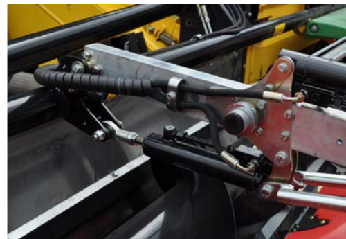
Installing the cylinder
